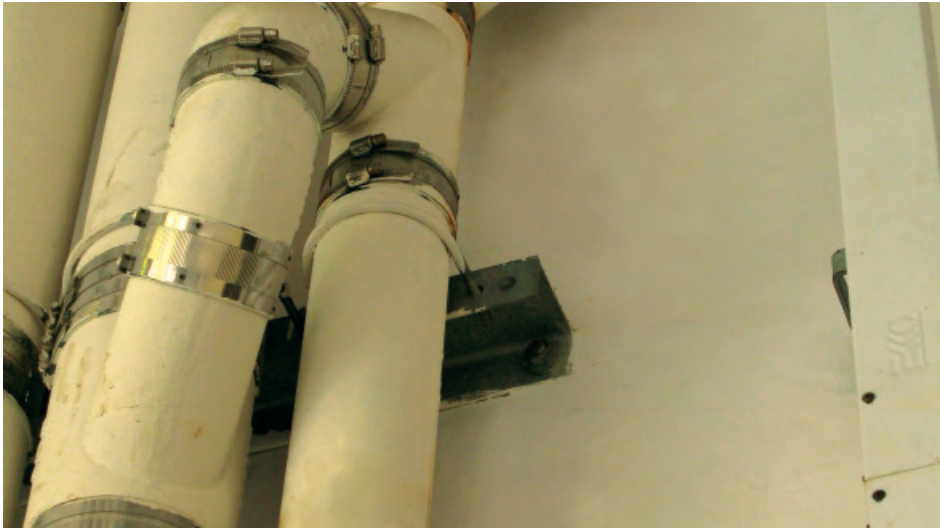
Securing Sewage Pipes
