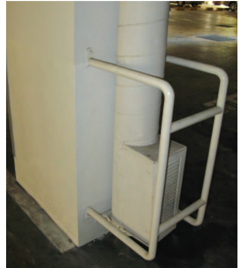
Securing Protecting Frames for Pipings
