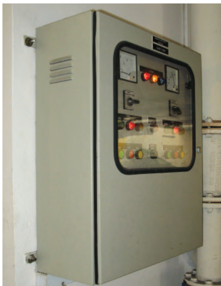
Securing Electrical Switch Box
