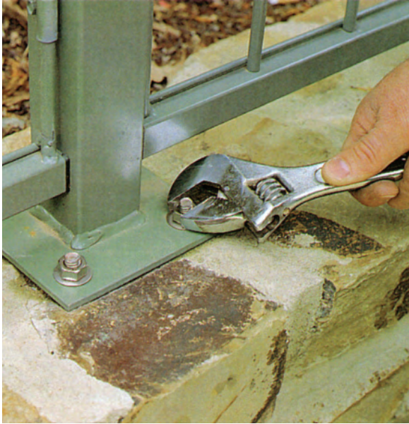
Installation of Railings
