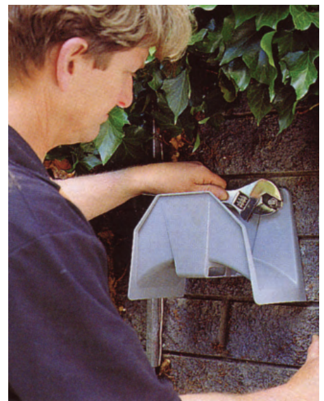
Fixing Brackets on Solid Bricks
